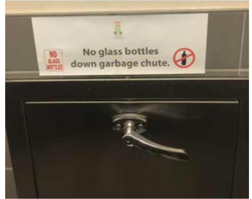
Trash chute features custom sign instructing residents against putting glass bottles down the chute.
